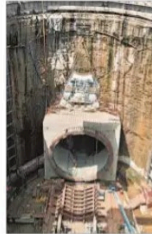
TBM assembly begins at Vikhroli in Mumbai. NHSRCL
